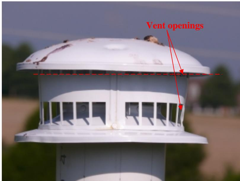
**Figure 4 – Close-up of GAS VENT station.**
